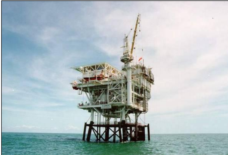
Kumul Oil Platform, Papua New Guinea
