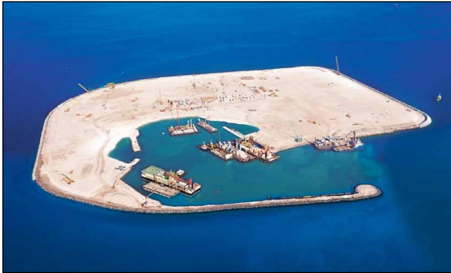
One of the Upper Zakum islands under construction
