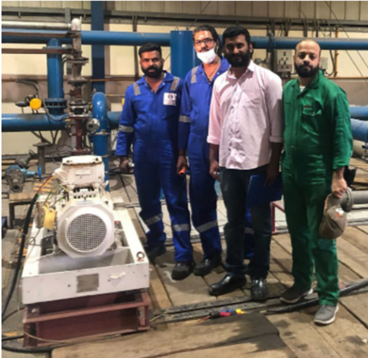
Engineers completing testing of a newly refurbished sodium hypochlorite dosing pump for ADNOC in the Amarithh UAE facility. (Image source: Amarithh Ltd.)
