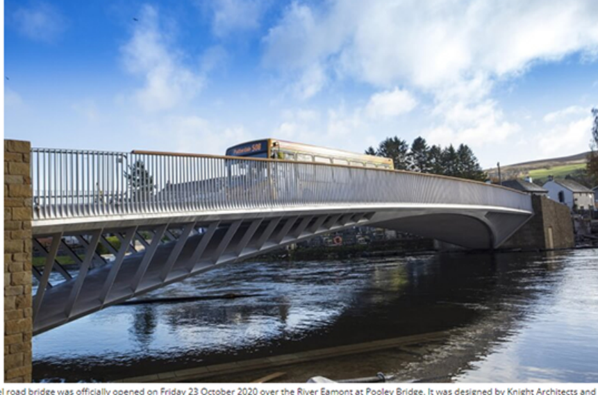
UK's first stainless steel road bridge was officially opened on Friday 23 October 2020 over the River Eamont at Pooley Bridge. It was designed by Knight Architects and uses duplex supplied by Outokumpu. Photo Courtesy of Outokumpu.
