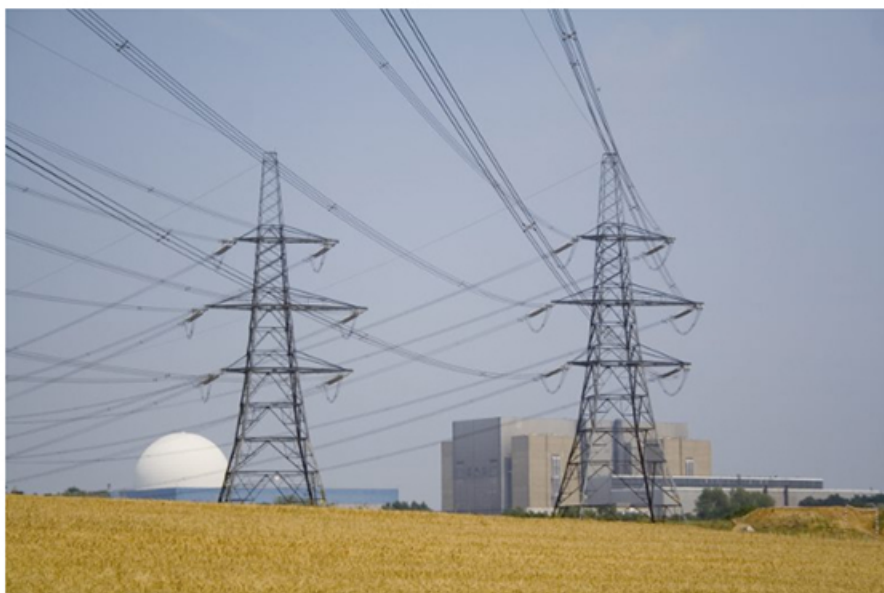
Sizewell Nuclear Power Station, Suffolk, England. (Image source: Amarith Ltd.)
